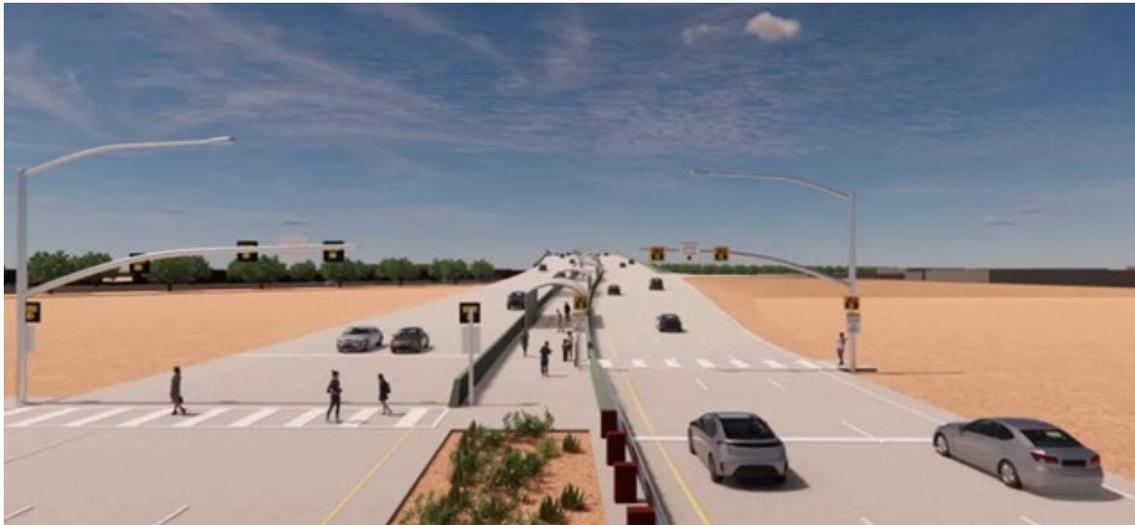
To access the center lane bikers and pedestrians would activate a HAWK light, stop traffic and make their way to the center island. At the opposite side of the bridge they'd again activate a HAWK light and exit to the sidewalk/bike path outside of the roadway. It's the only such design I've ever seen, and it has caused some considerable push back from the community.
